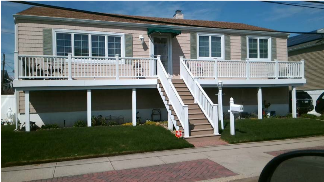
Figure 15: Elevation of structures has been adopted by approximately 20% of the buildings inspected since the effects of Super Storm Sandy in 2012.
